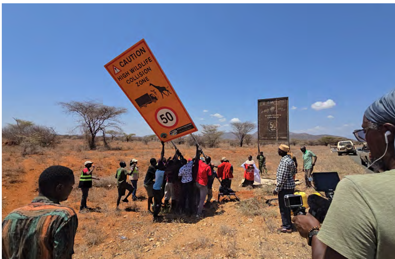
Installation of wildlife awareness signage along the A2 highway
